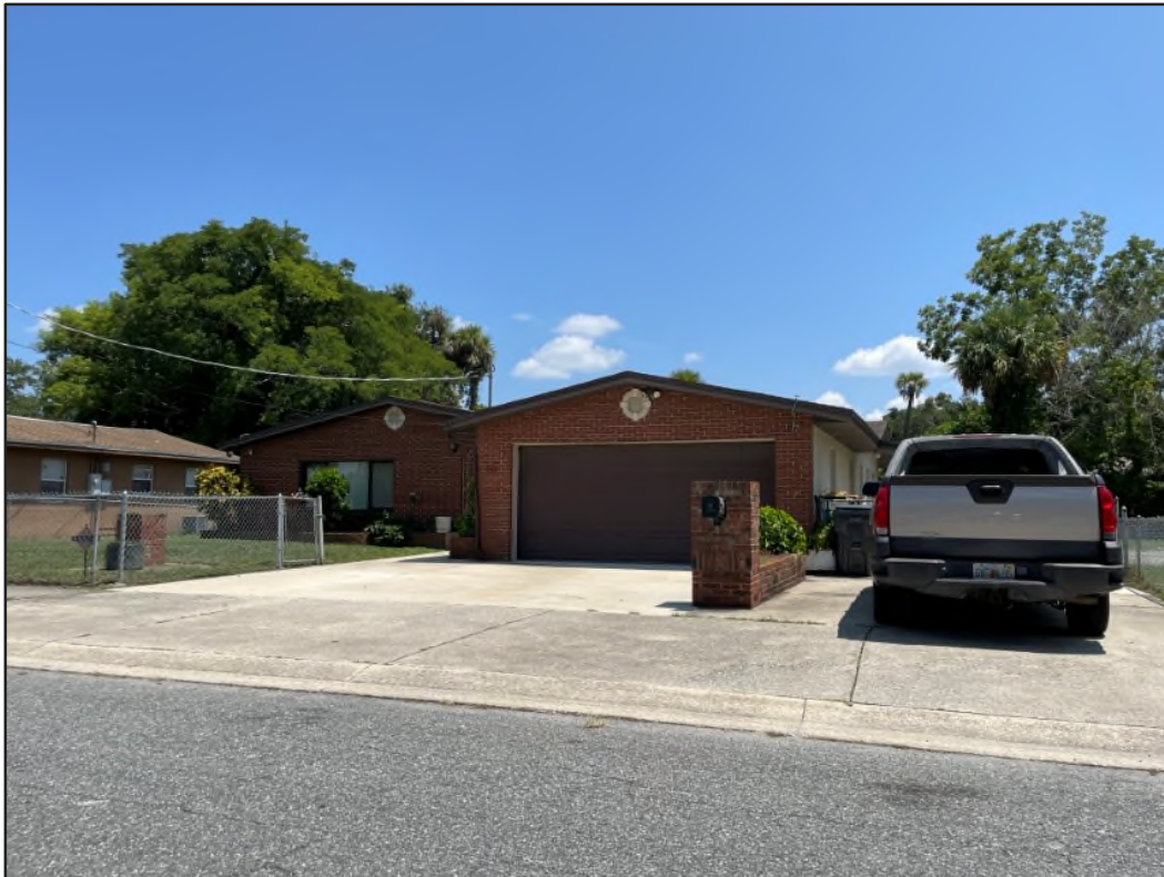
Figure 55. Lawson House at 945 Wager Avenue.
