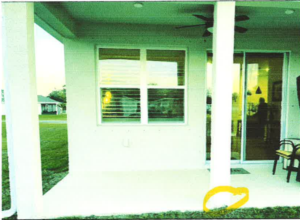
Beam in middle of patio
