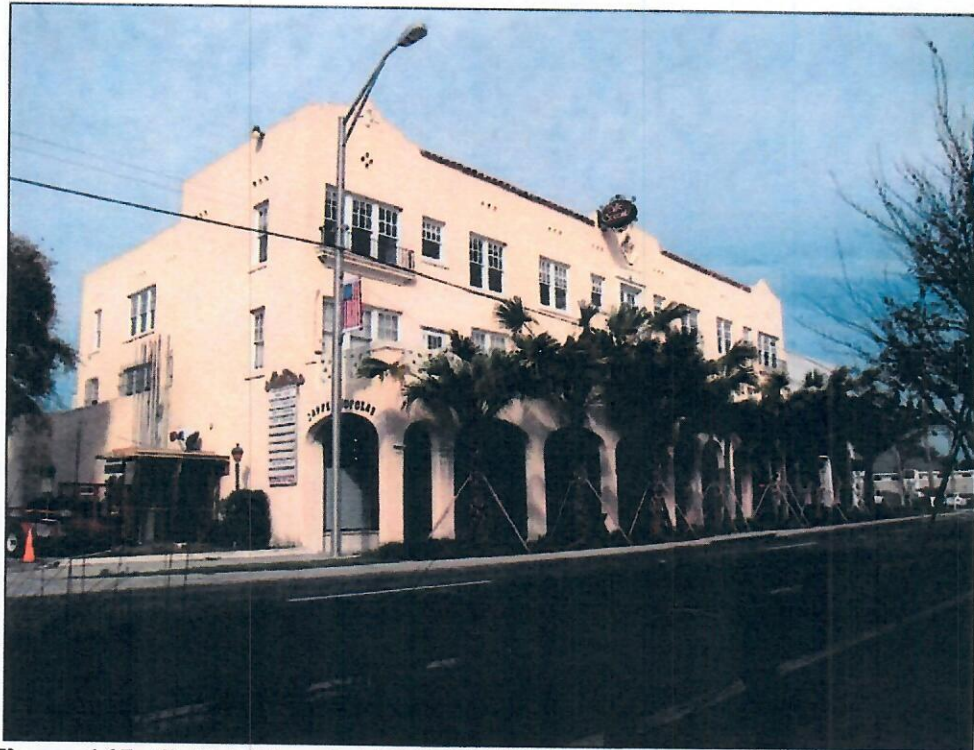
Figure 145: Caffè' Chocolat/ 302-310 S Washington Avenue (8BR514), facing northwest
