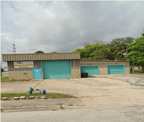
400 Garden Street Vacant Building – Before
