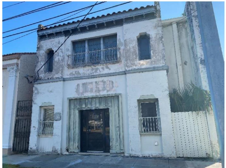
Figure 34. Dilapidated Historic Building
