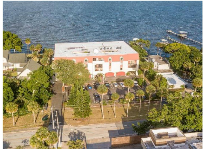
Figure 9. Existing Multi-Family Housing
