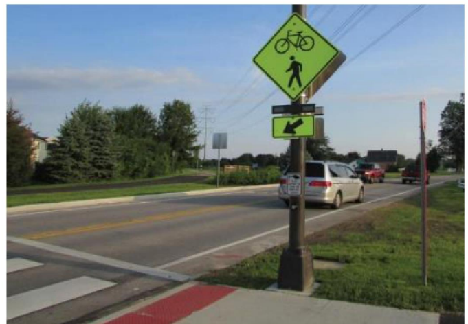
Figure 19. Activated Crosswalk Flash
