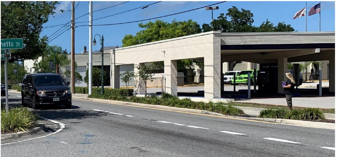
Figure 45. Pedestrian Waiting at Unmarked Crosswalk
