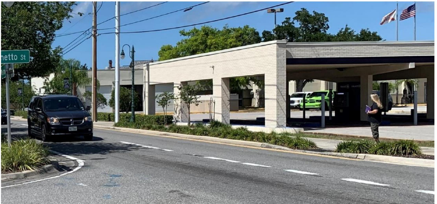
Figure 45. Pedestrian Waiting at Unmarked Crosswalk
