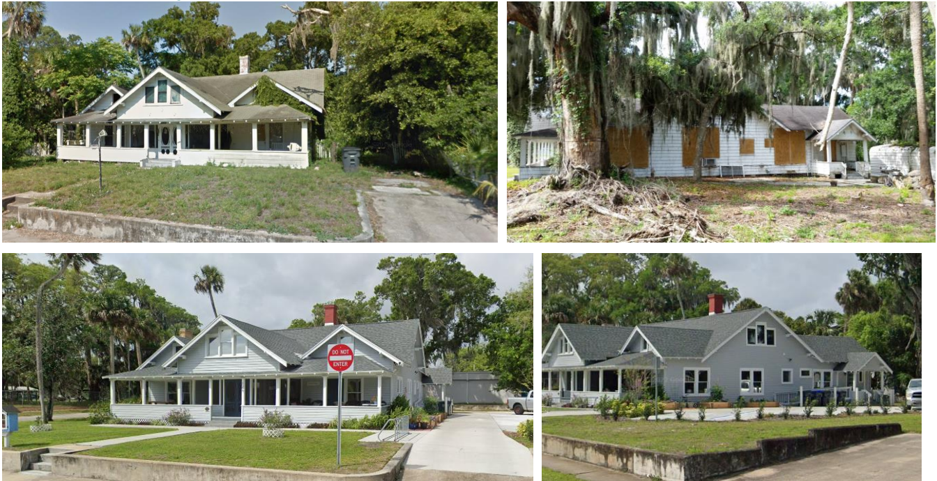
Figure 5: East-Façade - Main Entrance (2016 & 2025)
