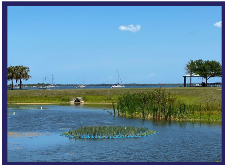
Figure 4. Floating Treatment Wetland at Sandpoint Park
