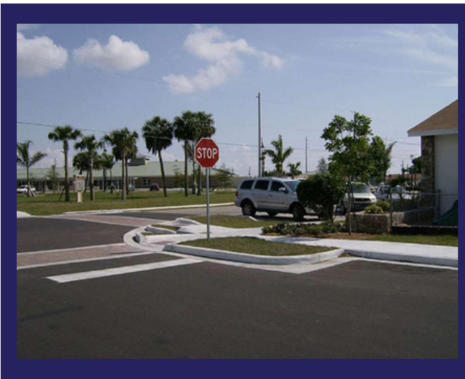
Figure 7. A corner extension slows vehicle turning speed
